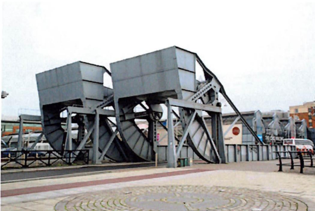
Figure 1. Scherzer Bridges at Georges Dock
