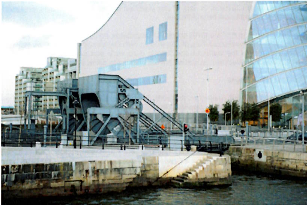
Figure 2. Scherzer Bridges at Spencer Dock
