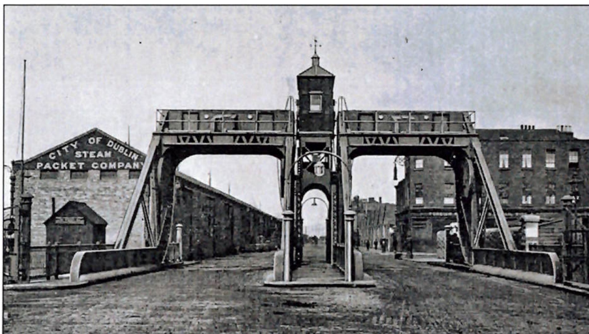
Figure 3. Spencer Dock bridges in 1913. Note the appearance of the pair of bridges as a single structure, reinforced by the central control cabin (Now removed).
