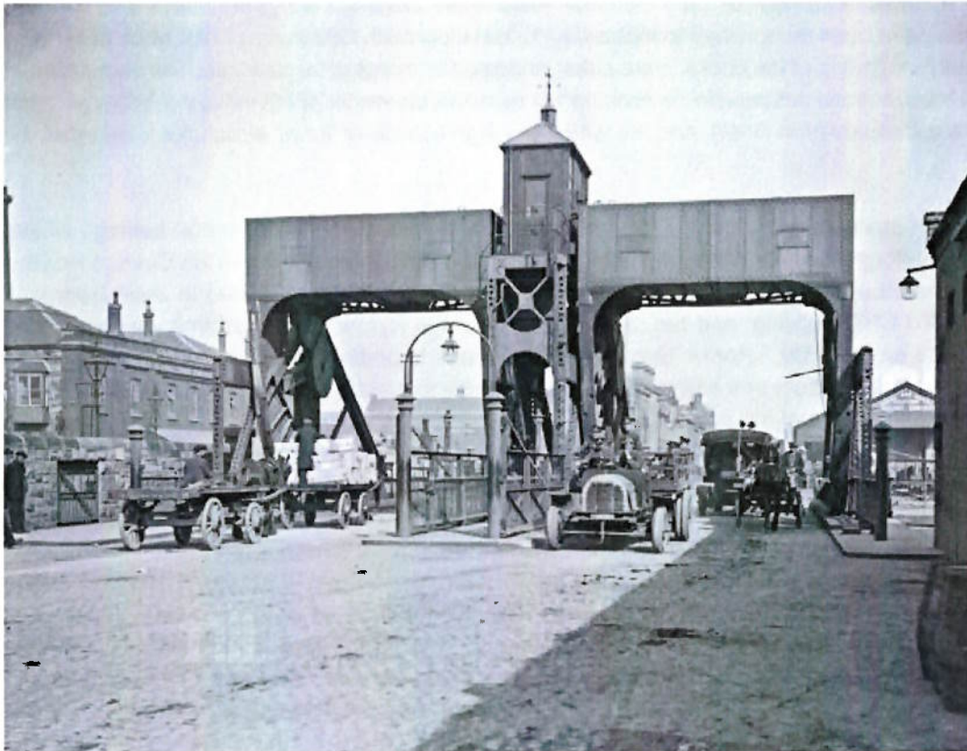
Image of Scherzer Bridges on North Wall Quay from the Lawrence Collection (National Library of Ireland)
