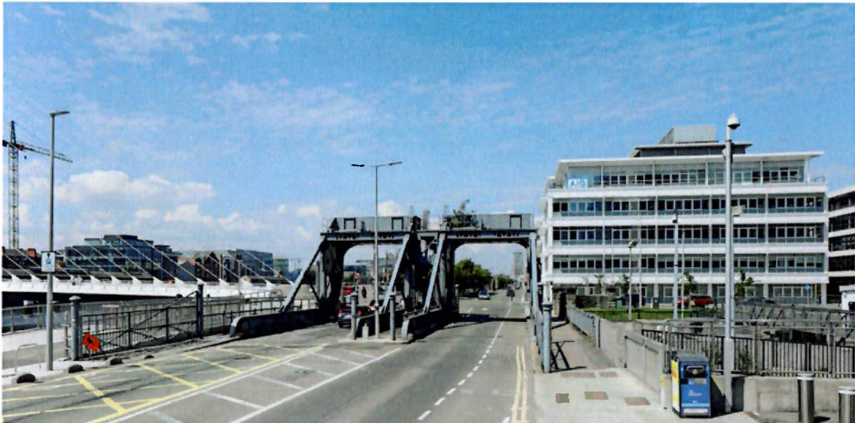
Figure 5. Current appearance of Spencer Dock bridges.
